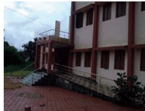
New Hostel Building
