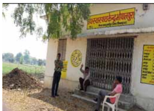
Poor cleanliness - cow dung being dumped adjacent to the SC building Bhopalpura (Dist:Tikamgarh)
